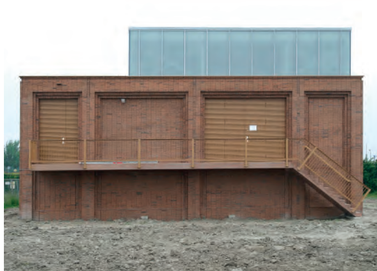
50 kV station Middelharnis
